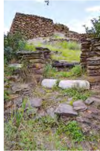
Detail of the use of greywacke for the construction of the Old Castle
