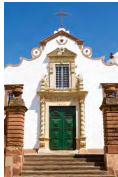
Main façade of Church of São Bartolomeu de Messines
